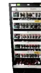
BATTERY TESTING SYSTEM
